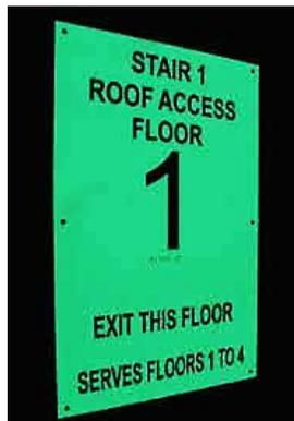
The International Fire Code sets forth minimum requirements for maintaining the life safety of building occupants. In this instance, stairwell identification signs are required at each floor landing in new and existing buildings with interior exit stairways and ramps connecting more than three stories. The intent of this requirement is to make signs visible and immediately recognizable to building occupants and emergency responders using the stairway.
