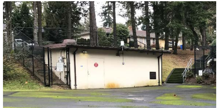
Cherry Crest pump station
