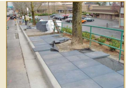
**Rubber sidewalk panels at NE 10 St west of 102 Ave NE allow tree roots to grow under the sidewalk without creating a trip hazard.**
